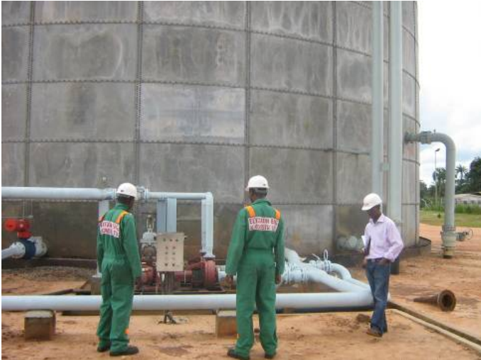
De-sanding / Desludging of 25,000 barrel Crude Oil storage Tank, at Addax Izombe Flow Station
