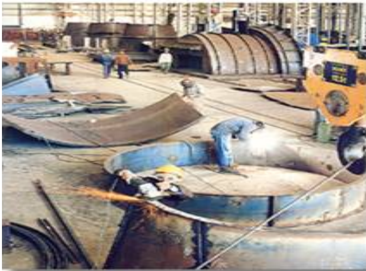
Figure 1 API 650 STORAGE TANK ERECTION
