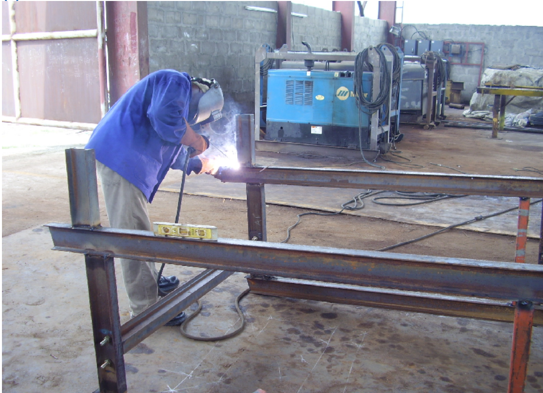
Above: Steel Structural Fabrication of Canopy structures for Addax Petroleum (b) below, commissioning of line heater Auto Ignition system at Addax Izombe flow Station
